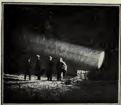
Powerful searchlight for illuminating hangars.
