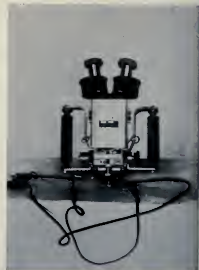
Fig. 19. Apparatus for seeing wireless signals.
