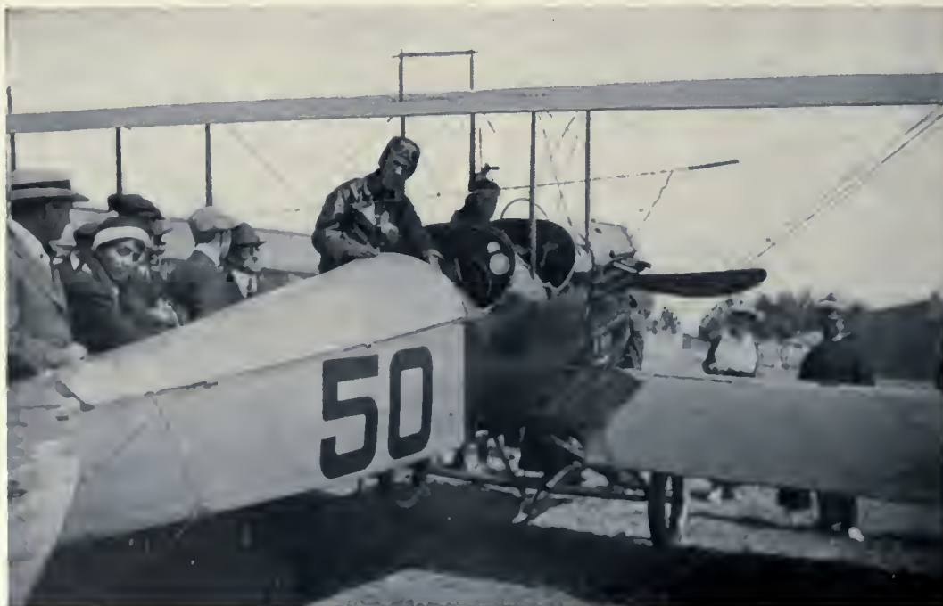
U. S. Army Aeroplane No. 50 of the North Island aviation school which was one of the aeroplanes which was equipped by Capt. C. C. Culver for radio work, the aerial wires being shown above the upper plane in the picture. Lieut. Herbert Dargue, U. S. A., is seen at the pilot's wheel, while Major Frank P. Lalm is in the observer's seat. The officers had just completed a flight.
